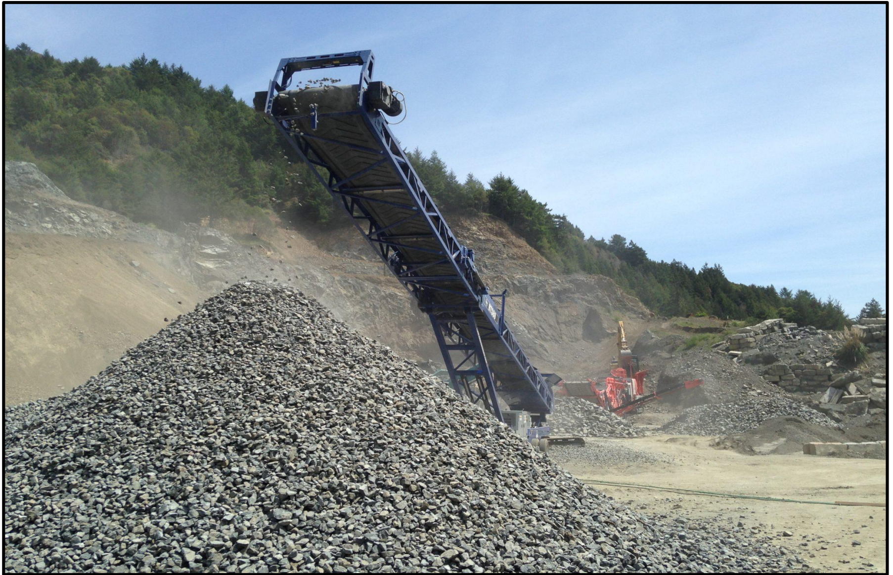
High Conveyor Drop
