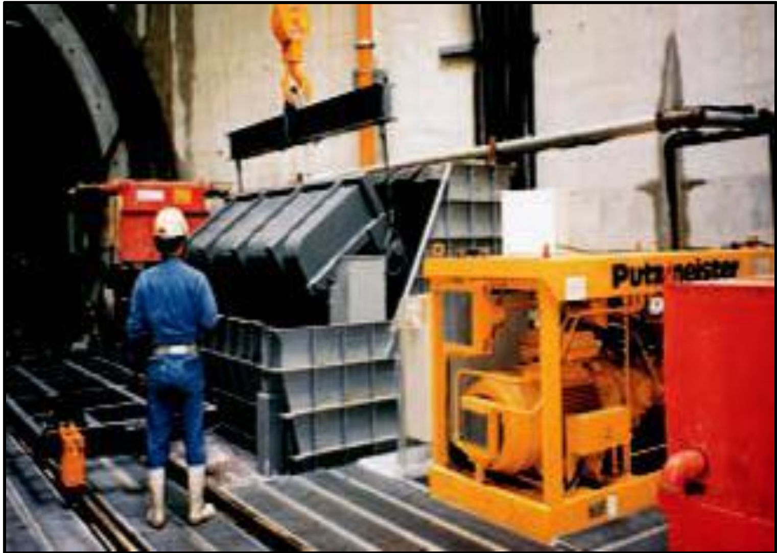
Transfer of muck in a shaft, construction site
