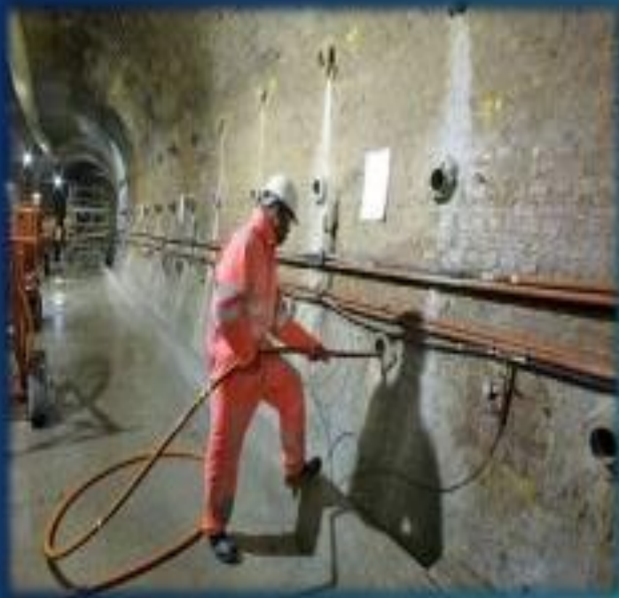
Guniting in tunnel
